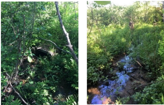
24 inch wooden culvert input
