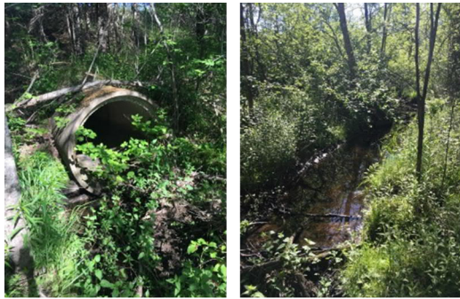
48 inch outflow culvert
