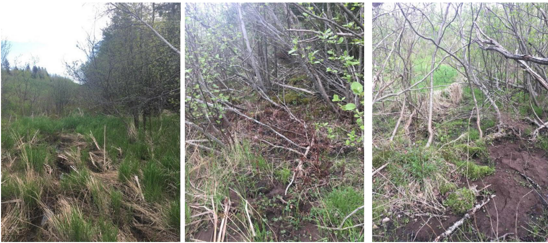
Culvert for WC-13B:
